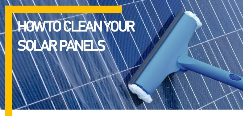
Solar Panels are generally self cleaning, but in particularly dry areas or where panel tilt is minimal, dust and other substances such as bird droppings can build up over time and impact on the amount electricity generated by a module. Grime and bird poop doesn't need to cover an entire panel to have an effect. This is where cleaning solar panels may have to be done.
